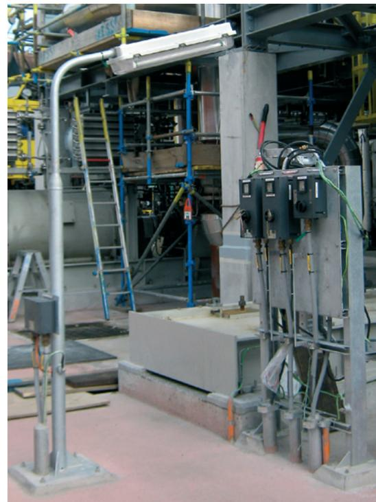
Schuch T8 fluorescent fittings include a strong internal steel sleeve for easy pole mounting
